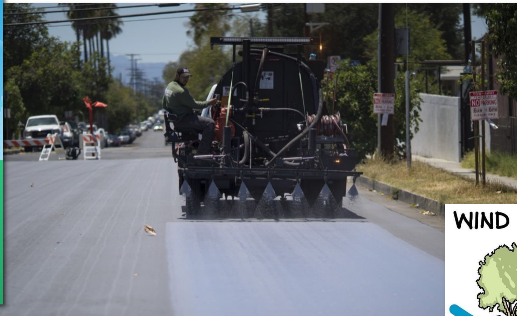
A worker applies a reflective pavement coating to a street in the Pacoima area of Los Angeles on July 19. Photographer: Eric Thayer/Bloomberg
